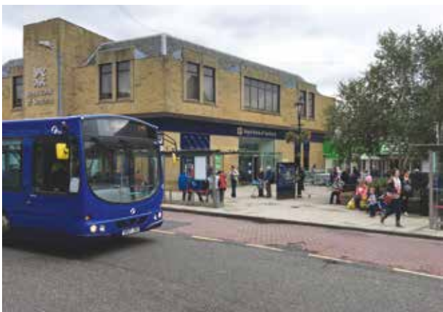
Newmarket Street Bus Station
