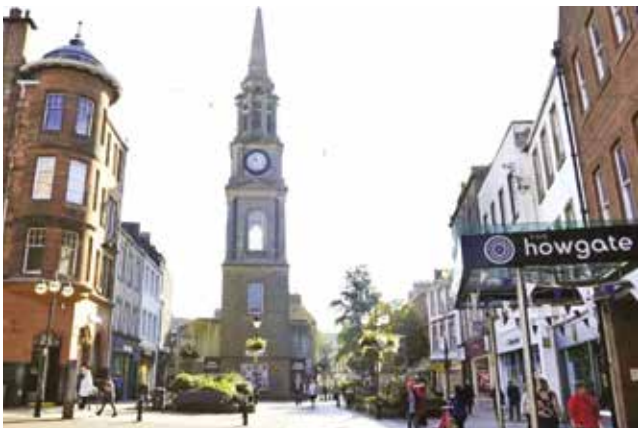
From the High Street main entrance
